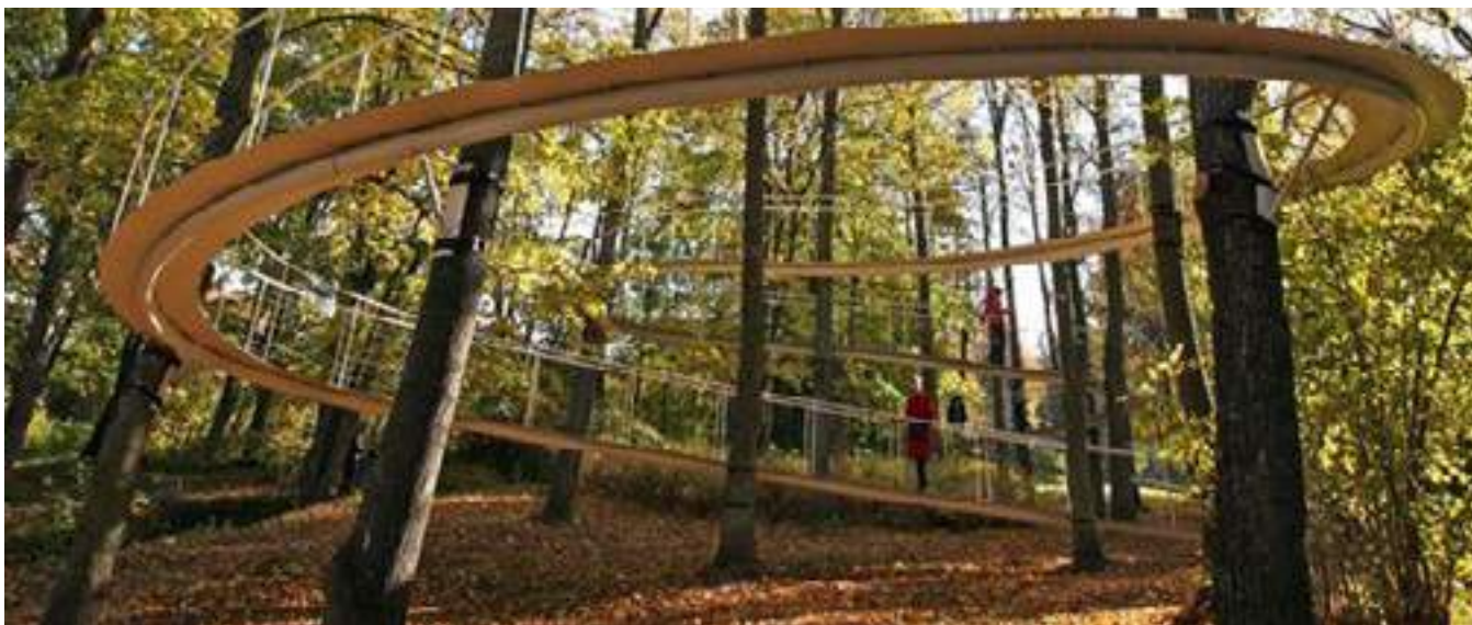
A Path in the Forest (Estonie) - Transsolar & Tetsuo Kondo Architects
